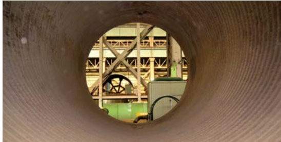
Reactor Vessel Soudotape 309L Q5 + Record 6/74 Q5
